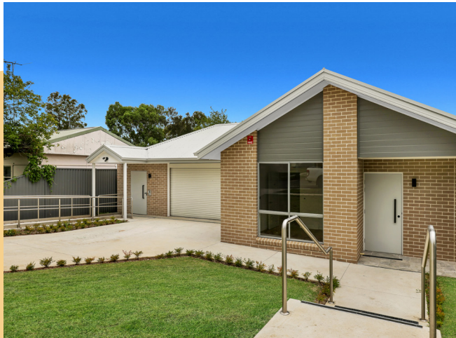
Internal/external ramp access
